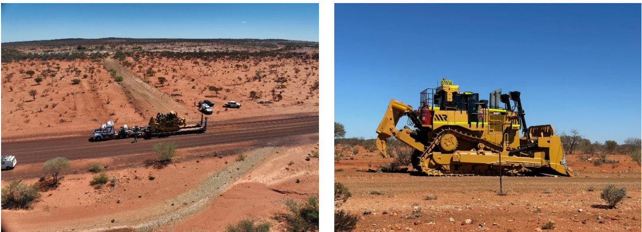
Figure 2 - Mobilisation to site and site preparation activities
